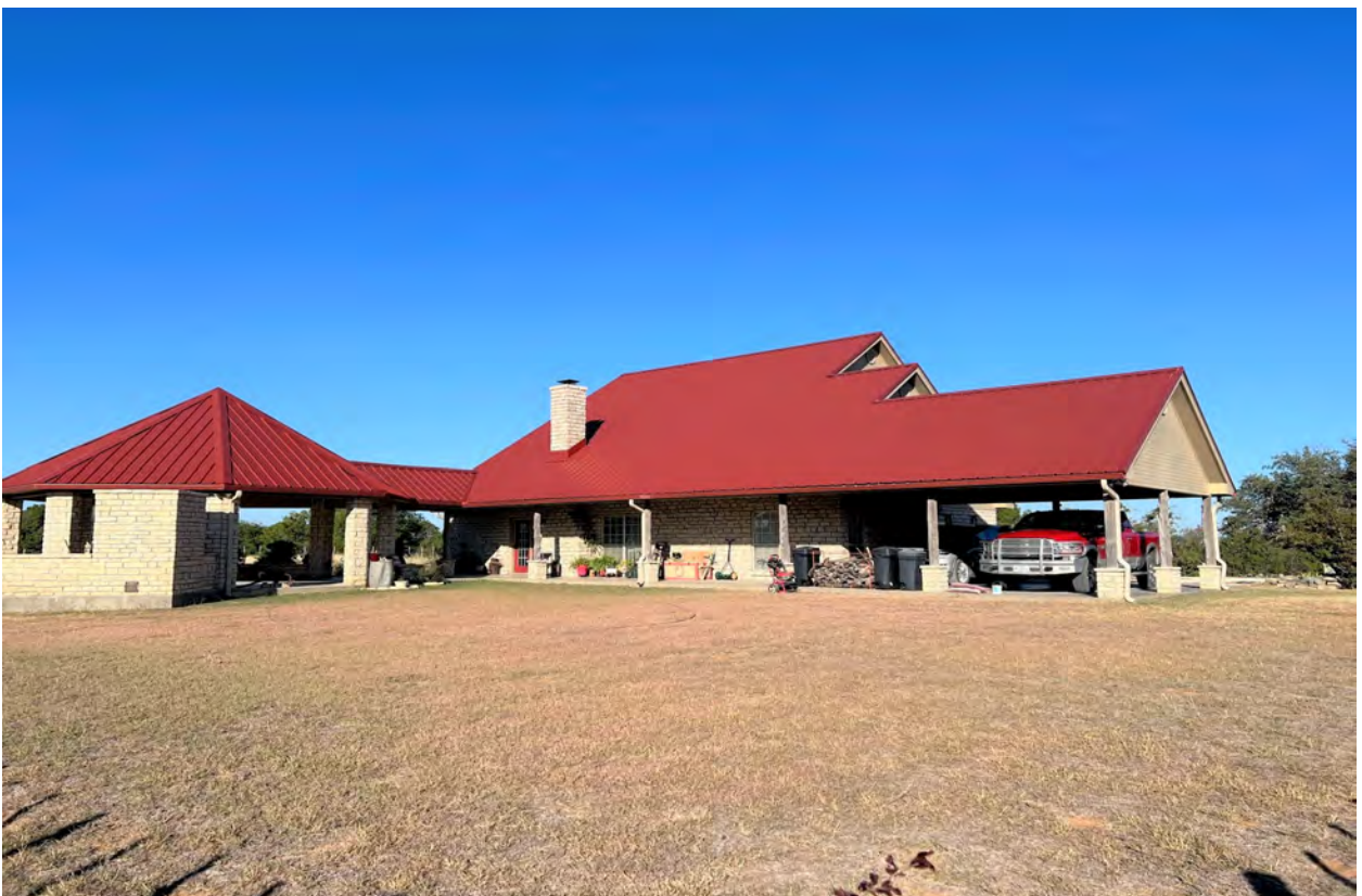
Rear/Overall View of Subject Dwelling 10/19/2022 Interior View 10/19/2022
